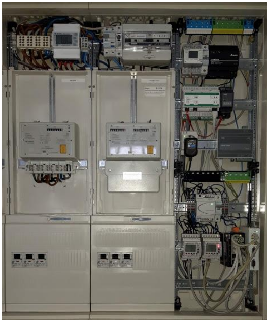
Figure 6: equipped central control box with Goflex components
