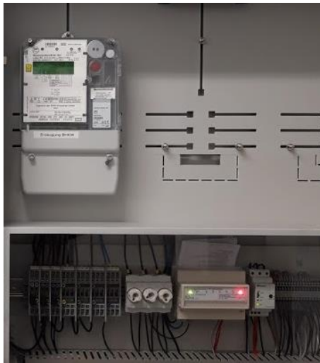
Figure 12: Measuring device with fibre optic relay
