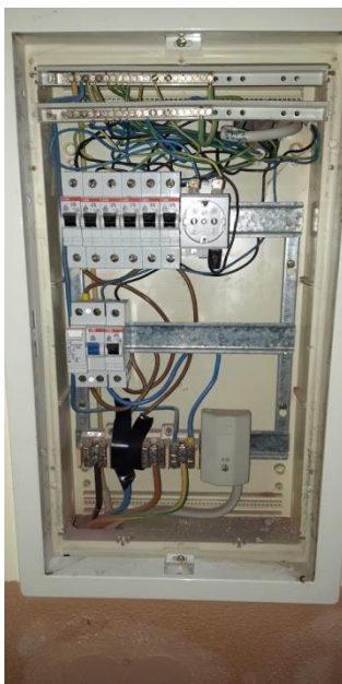
Figure 5: existing electrical sub-distribution on floor
