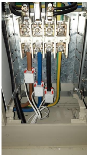
Figure 13: Instrument transformers
