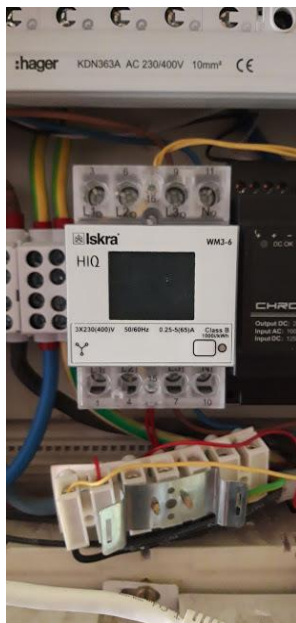
Figure 7: Z-Counter - Control cable connected
