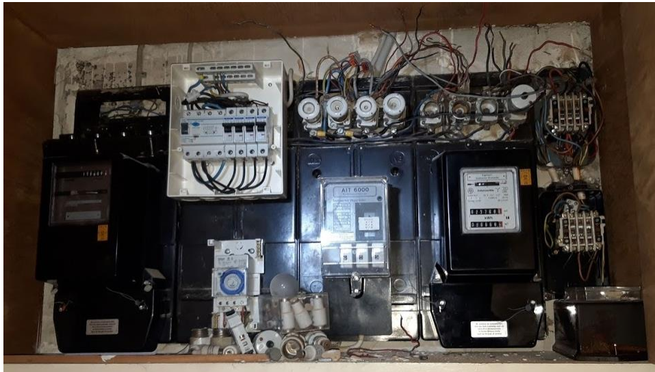
Figure 8: Old meter distribution
