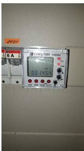
Figure 14: Top hat rail counter
